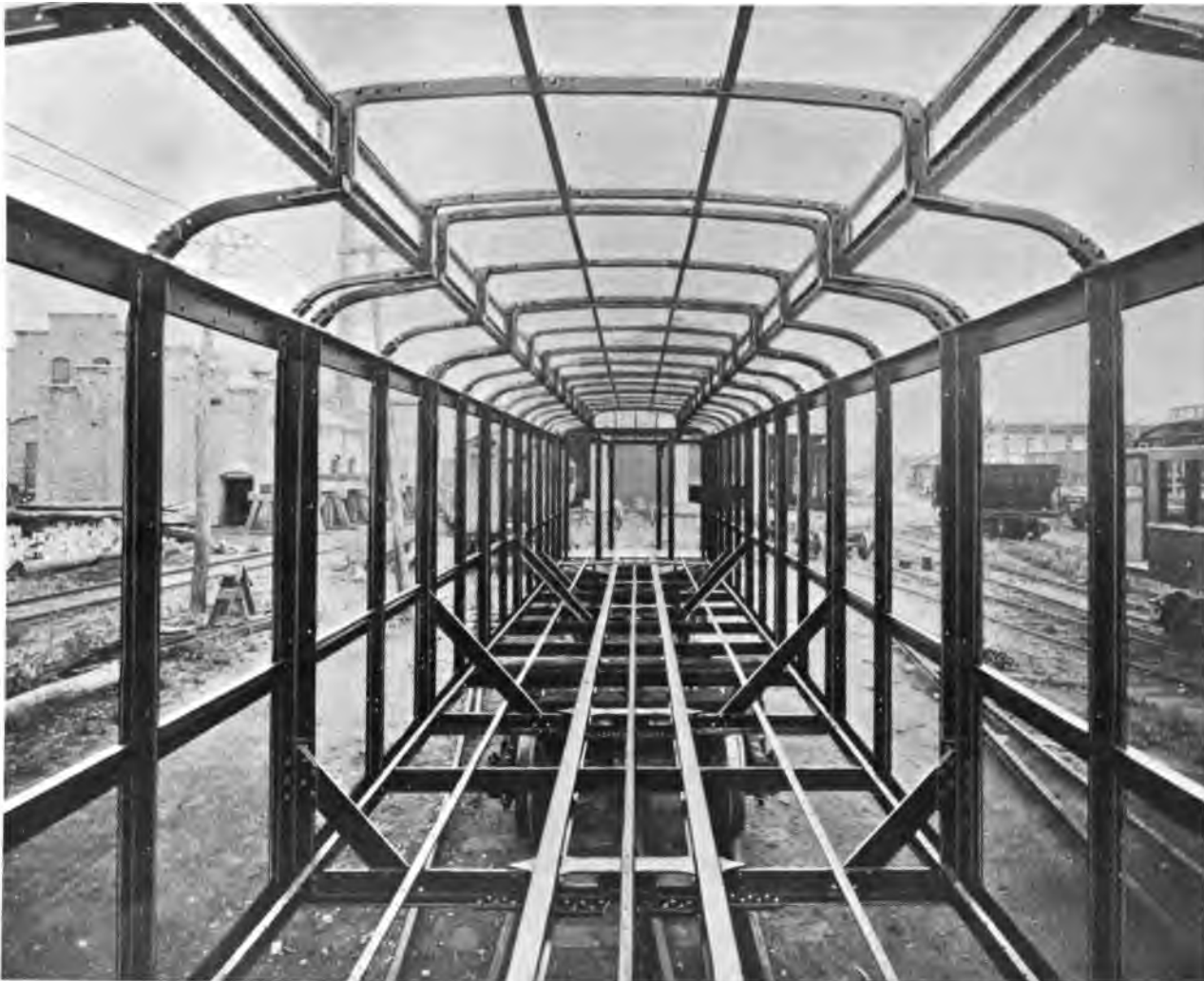
INTERIOR VIEW — SKELETON FRAMING OF STEEL CAR
